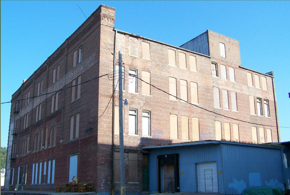
1888 Construction – Next to Railyard
