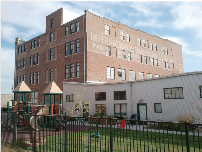
Above: Brownfield sites prior to redevelopment Below: Redeveloped Council Bluffs brownfield site
