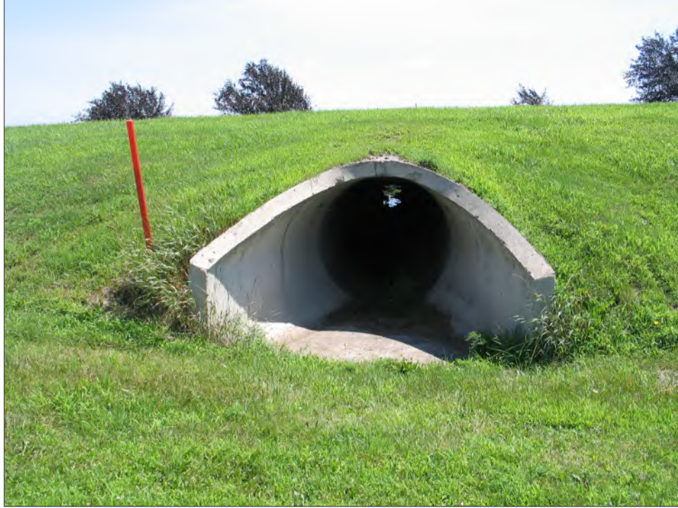
Figure 22. Example of a culvert in the project area. View to the east (7/15/25).
