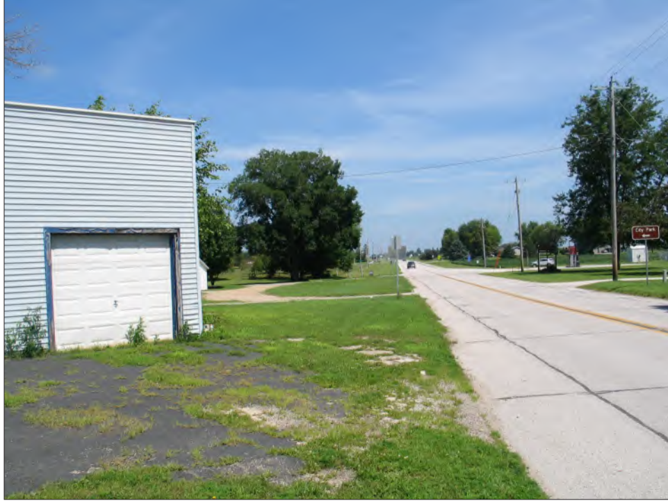
Figure 18. Water main replacement corridor at the intersection of Fitzpatrick and Sand streets. View to the north (7/15/25).
