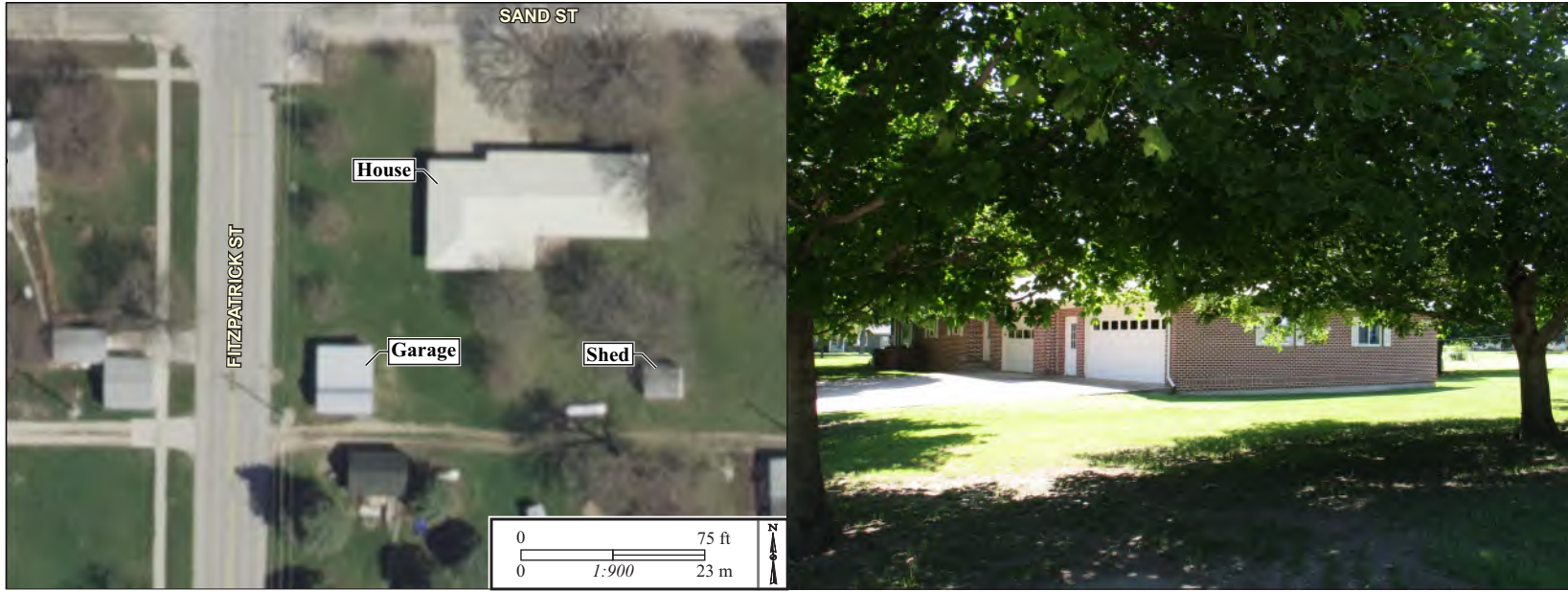
Figure 11. Property ID 8; Donald Karlovec Residence. View to the northeast (7/15/25).
