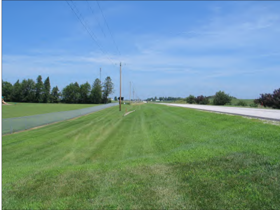
Figure 20. Water main replacement corridor at the intersection of Fitzpatrick and Adrian streets. View to the north (7/15/25).
