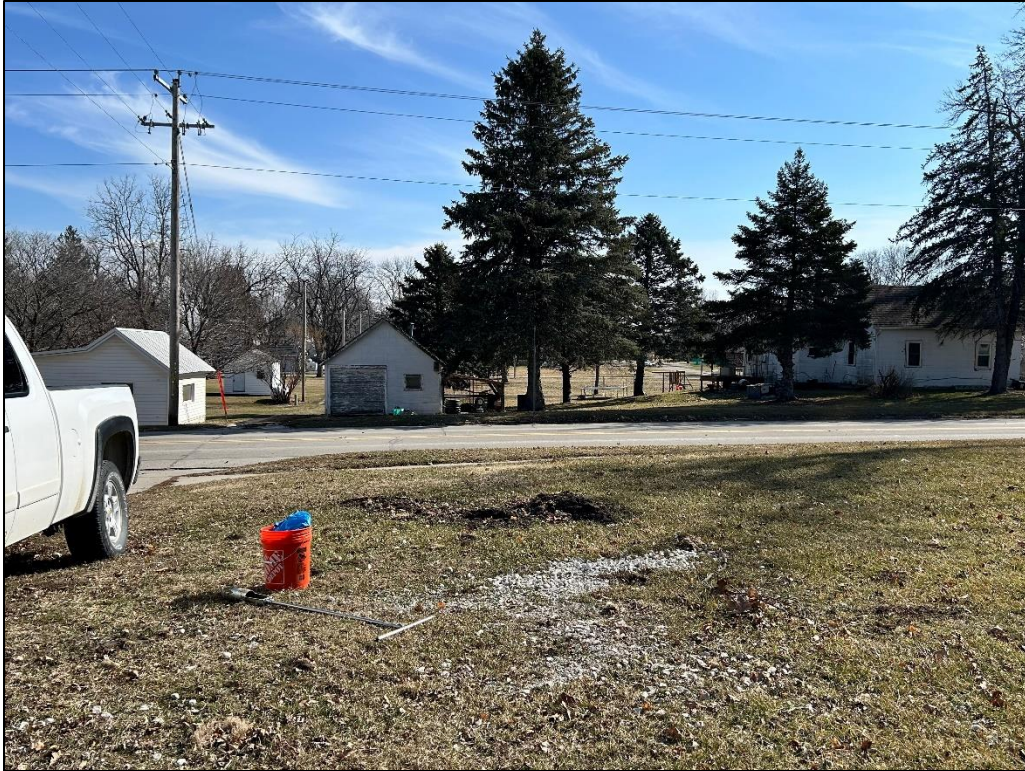
Figure 17: Project area overview facing south. Underground utilities located in this section.
