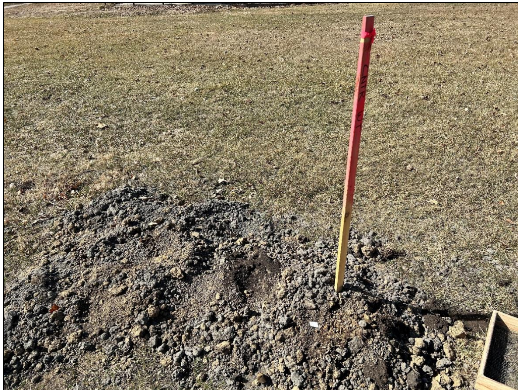
Figure 25: Overview of exposed soils and water tower location.
