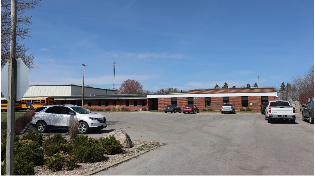
This photo was taken from the southwest side of the building.
