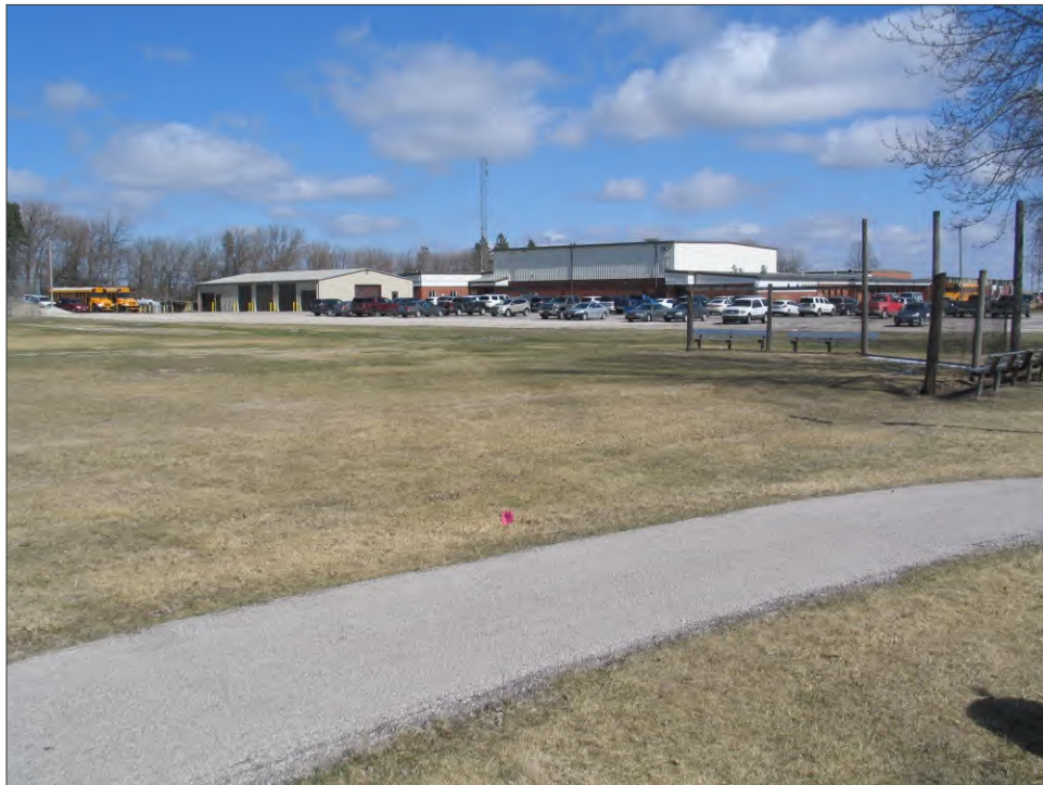
Figure 19. South portion of the project area. View to the northeast (3/11/26).
